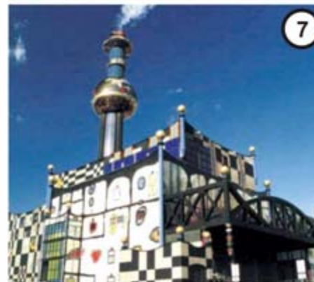
THE point of reference in the area: Incineration plant designed by the famous Austrian artist Friedensreich Hundertwasser
