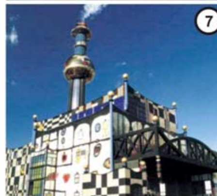
THE point of reference in the area: Incineration plant designed by the famous Austrian artist Friedensreich Hundertwasser
