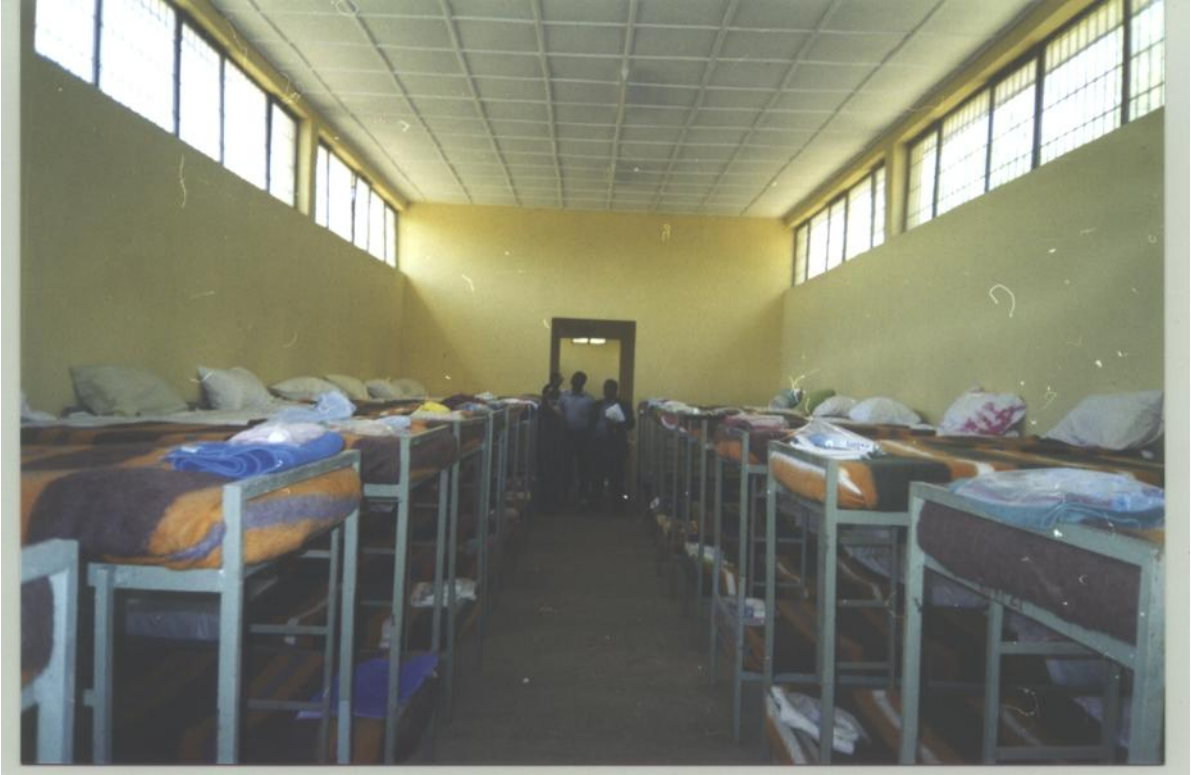
The new wing of the Diplo Prison built by Prisons Fellowship Ethiopia
